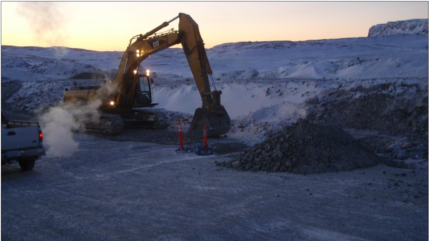
Photo 7: Cat 330 excavator tamping \frac{3}{4} crush on top of thermistor cables at chainage 1+30.
