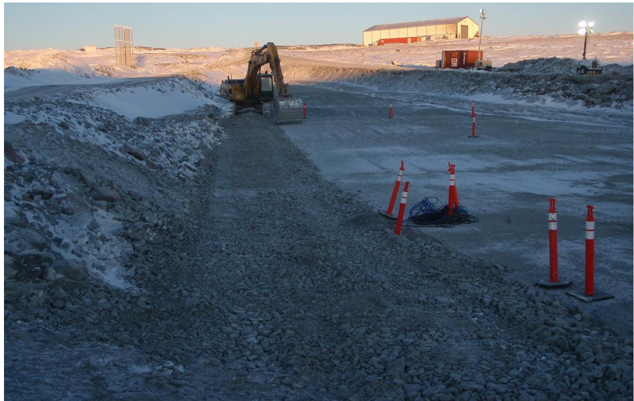
Photo 6: Transition material placed along the downstream side of the dam. Thermistor cables in foreground buried in a blanket of crush.
